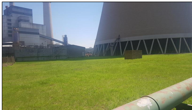
Figure 5 – Alternate view of the southern study area with one of the preexisting lime plants in the background.
