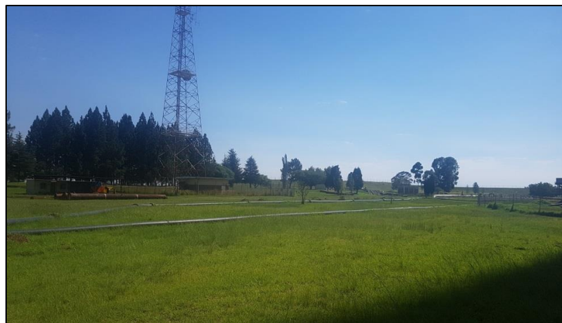
Figure 3 – View of the northern study area. Take note of the pipework above ground and ancillary infrastructure.
